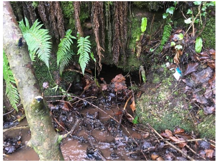
Watercrossing Structure W11
