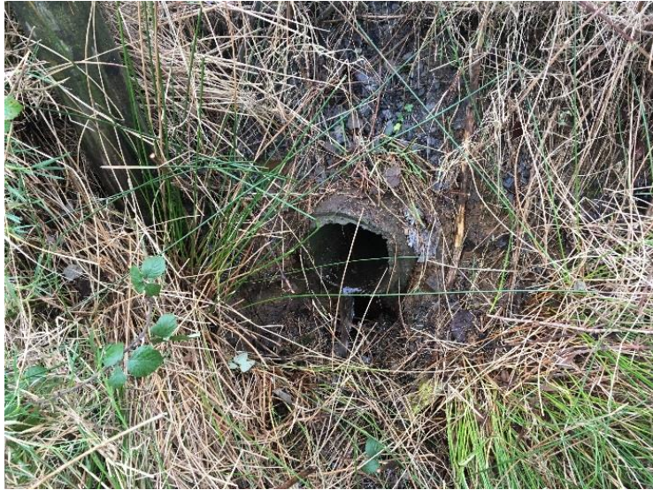
Watercrossing Structure W58
