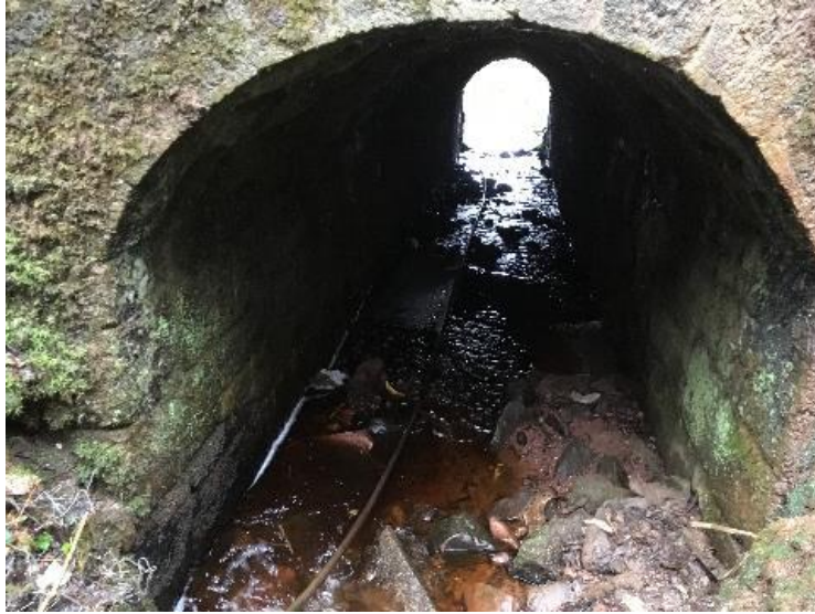
Watercrossing Structure W22
