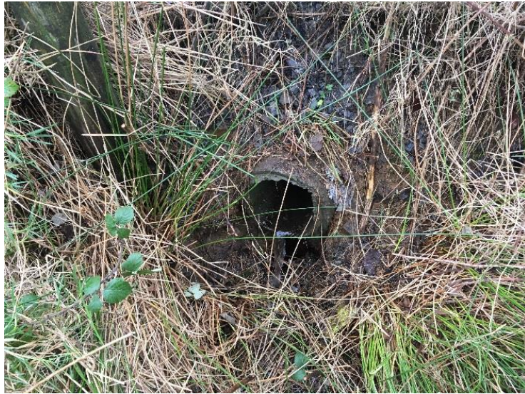
Watercrossing Structure W56
