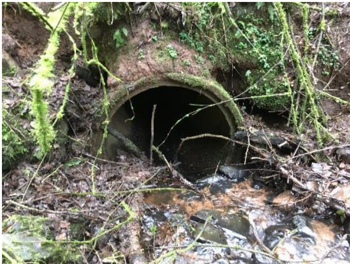
Watercrossing Structure W24
