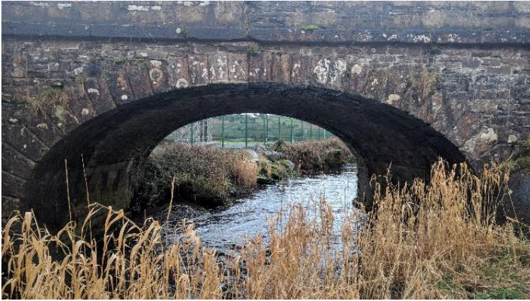
Watercrossing Structure W53
