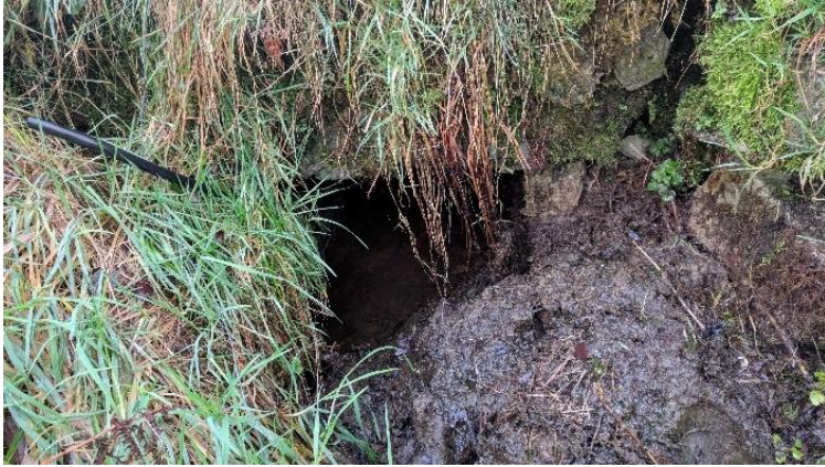
Watercrossing Structure W55
