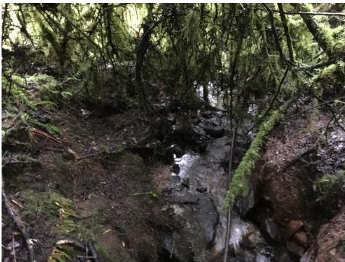
Watercrossing Structure W27
