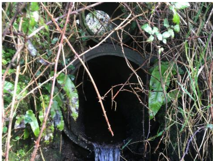
Watercrossing Structure W12
