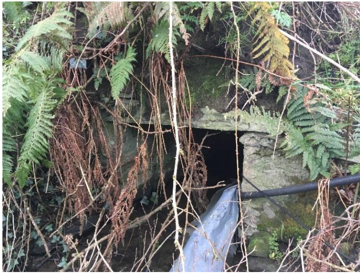
Watercrossing Structure W61
