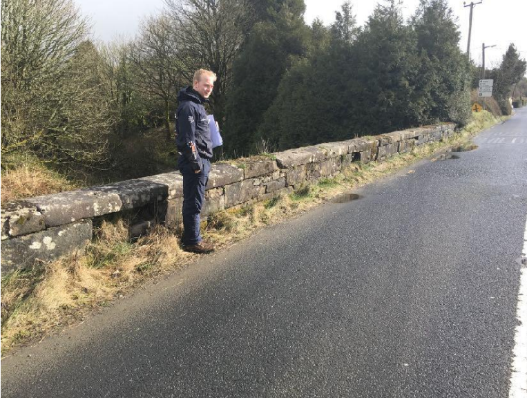
Figure 8: Showing the existing low parapet wall on Anglesey Bridge. Note lost ashlars
