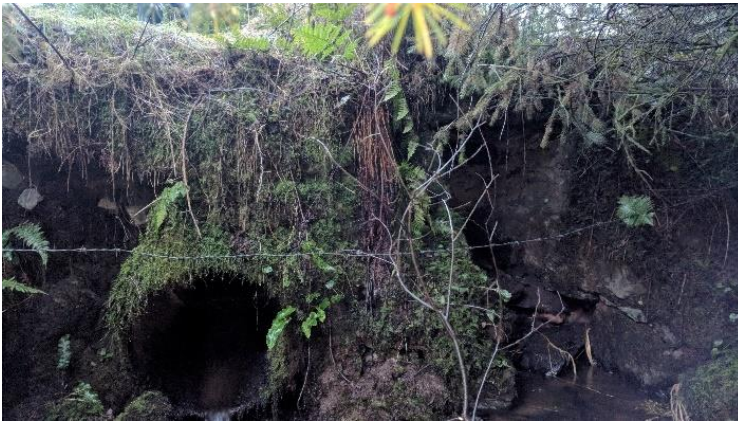
Watercrossing Structure W59
