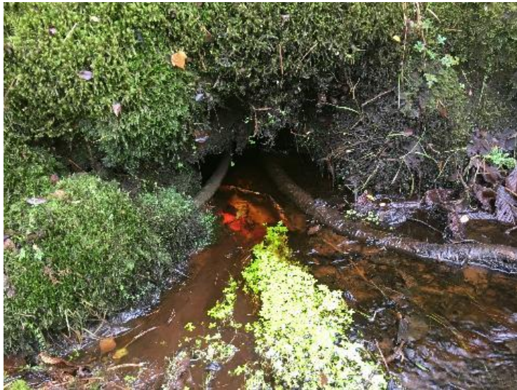
Watercrossing Structure W19
