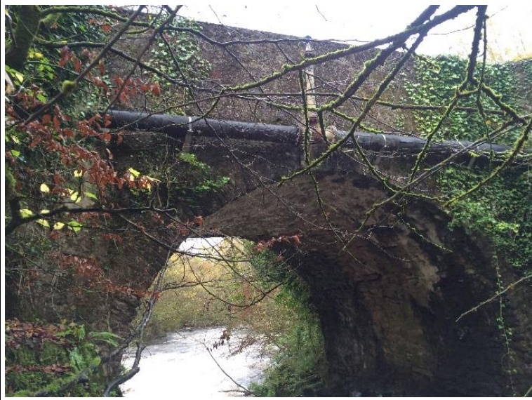
Watercrossing Structure W7
