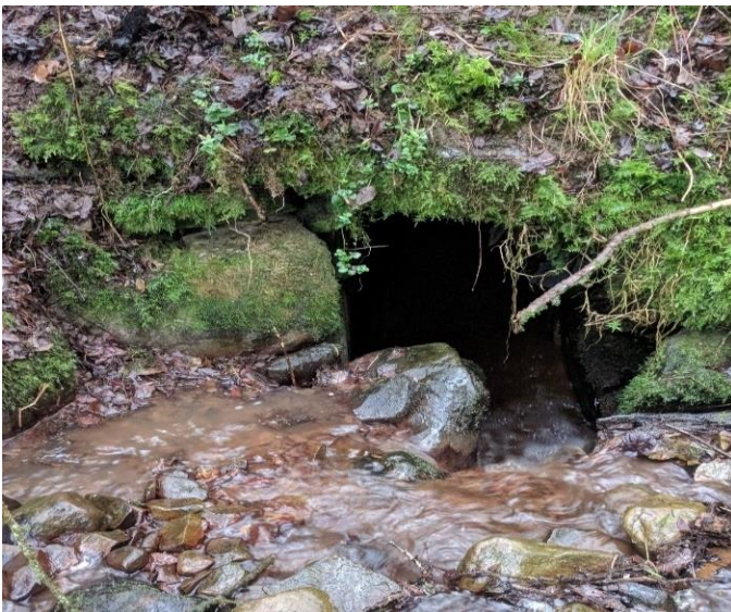
Watercrossing Structure W51
