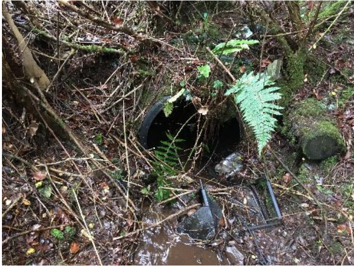
Watercrossing Structure W25
