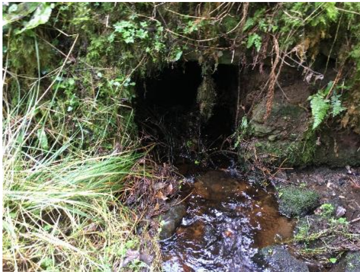
Watercrossing Structure W14
