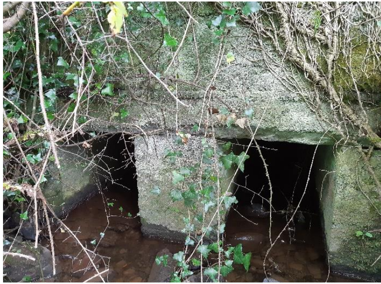
Watercrossing Structure W4
