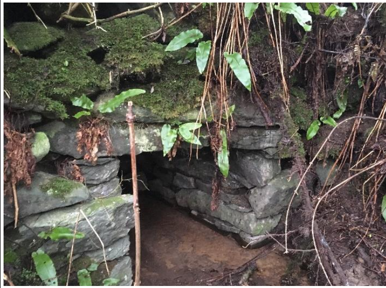
Watercrossing Structure W64
