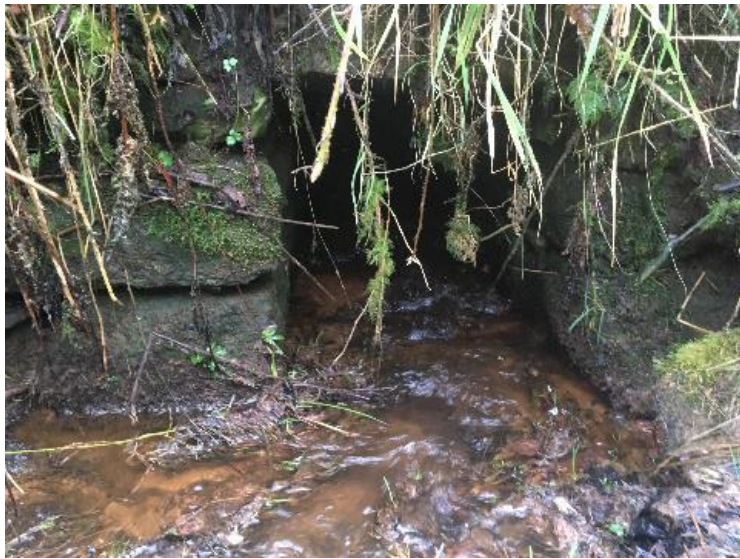
Watercrossing Structure W32
