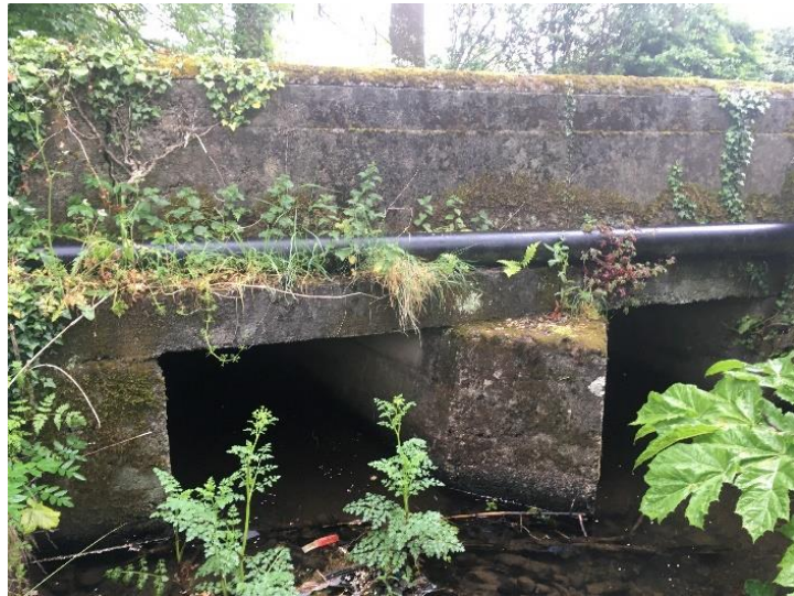
Watercrossing Structure W8
