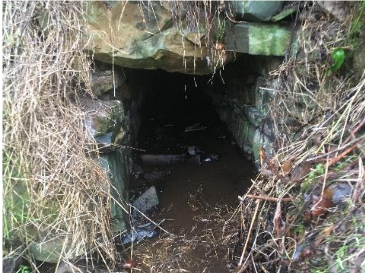
Watercrossing Structure W34
