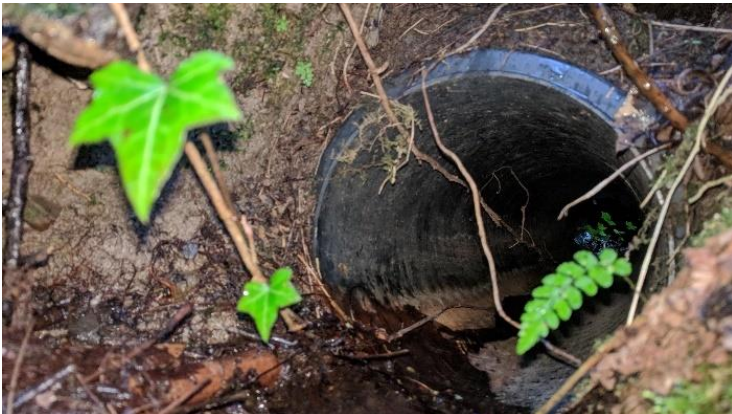
Watercrossing Structure W54
