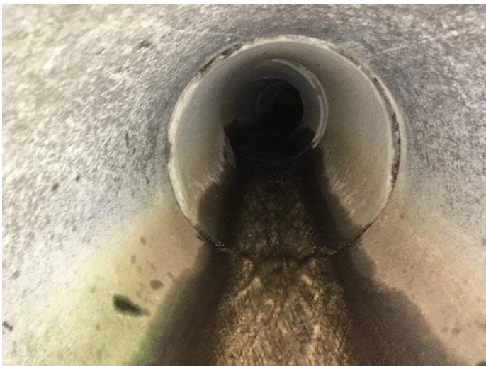
Watercrossing Structure W39
