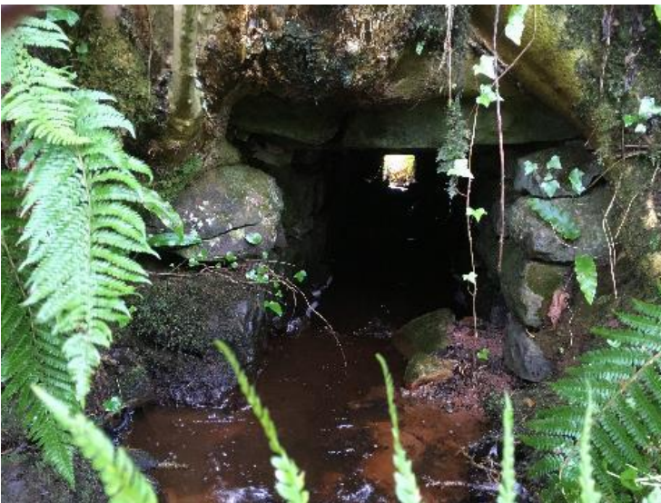
Watercrossing Structure W15
