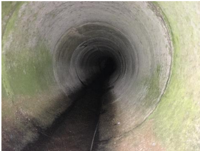
Watercrossing Structure W26
