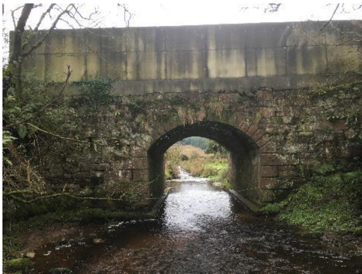
Watercrossing Structure W33
