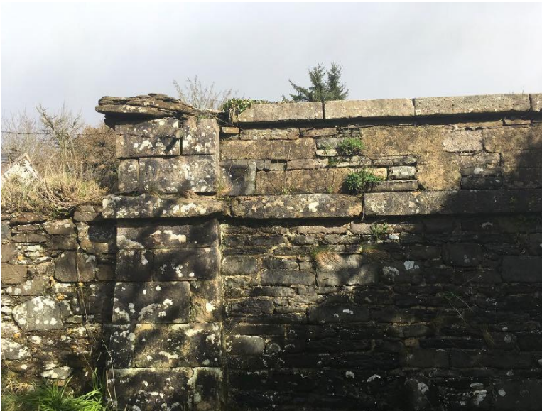
Figure 9: Showing the condition of the south western pier, note damaged coping stone
