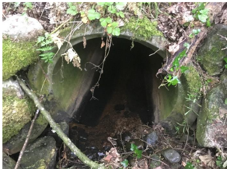
Watercrossing Structure W6
