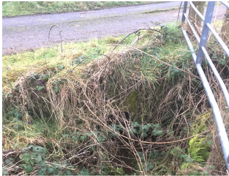
Watercrossing Structure W68
