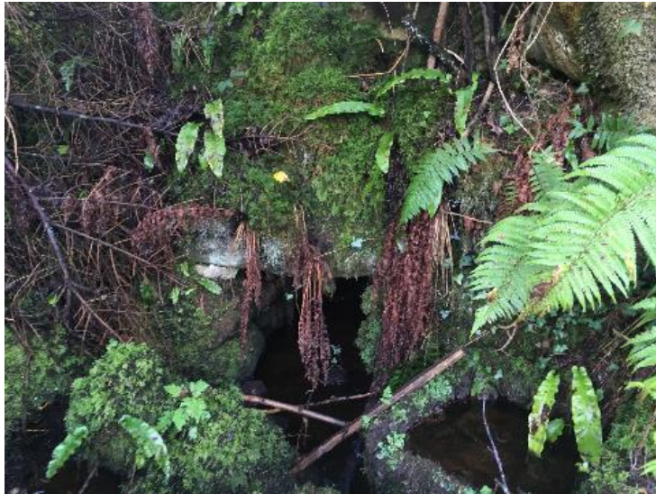
Watercrossing Structure W13
