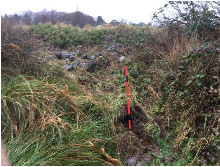
Watercrossing Structure W37
