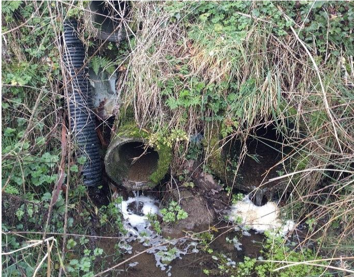
Watercrossing Structure W40
