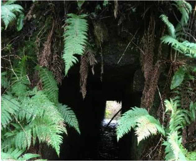
Watercrossing Structure W28
