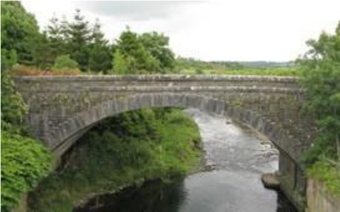
Figure 4: Goulburn Bridge Co. Limerick, shows similar design features to Anglesey Bridge (photo from NIAH Record 21904302) Note: Stepped voussoirs, the similar string course and the coping stones
