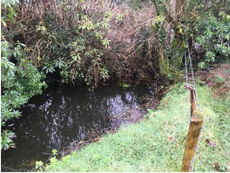
Watercrossing Structure W16
