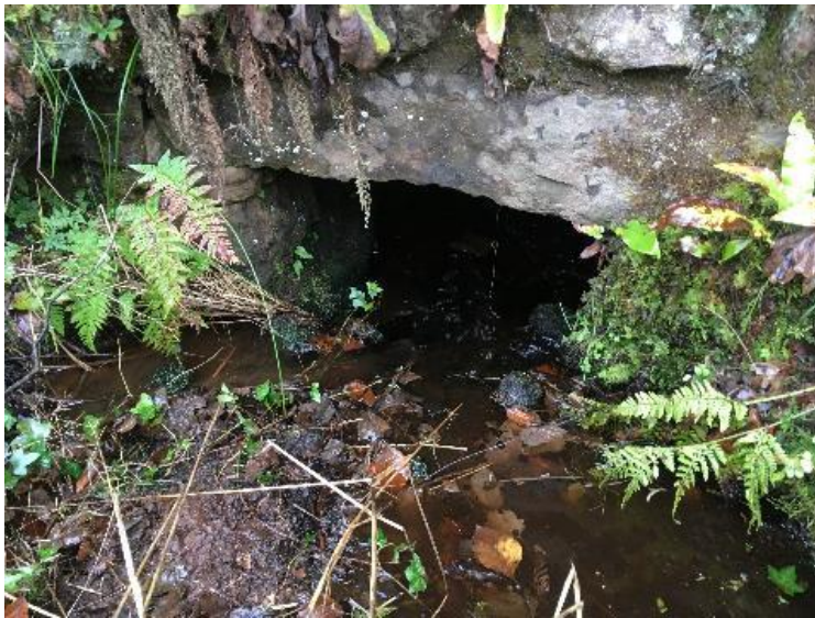
Watercrossing Structure W20
