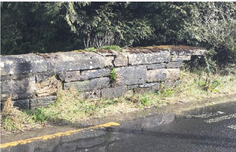
Figure 10: Detail of north eastern end of parapet, note loss of stones
