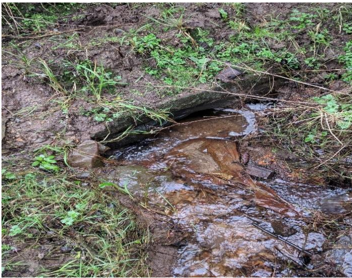
Watercrossing Structure W42
