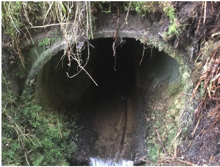
Watercrossing Structure W65
