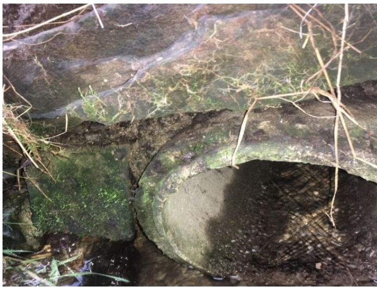
Watercrossing Structure W66
