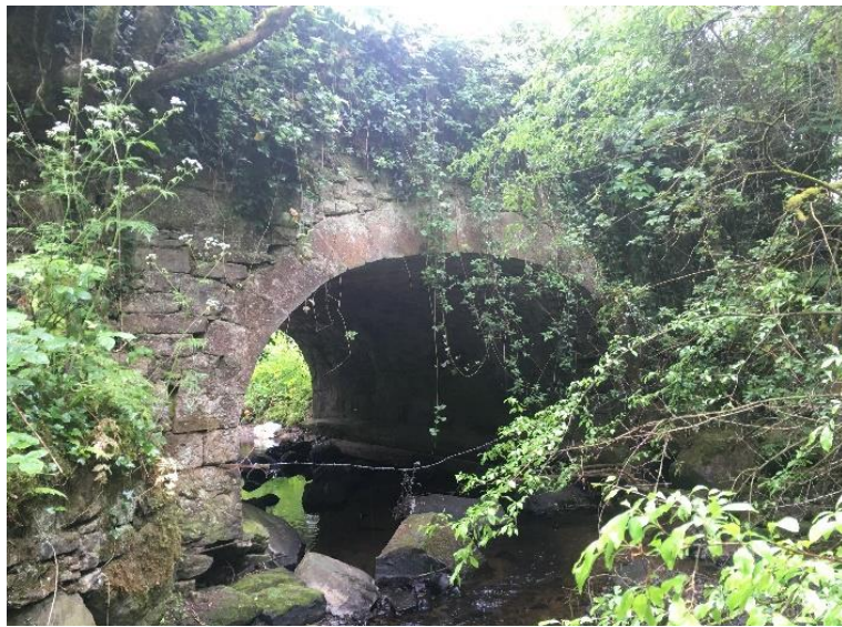
Watercrossing Structure W5
