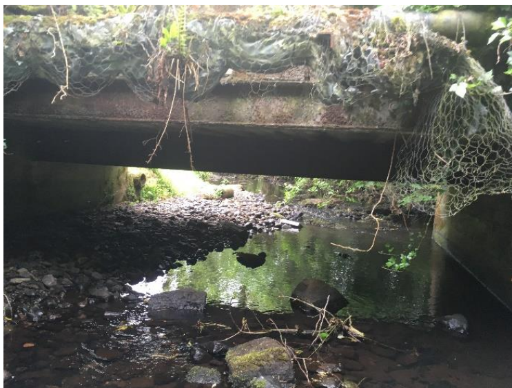
Watercrossing Structure W9
