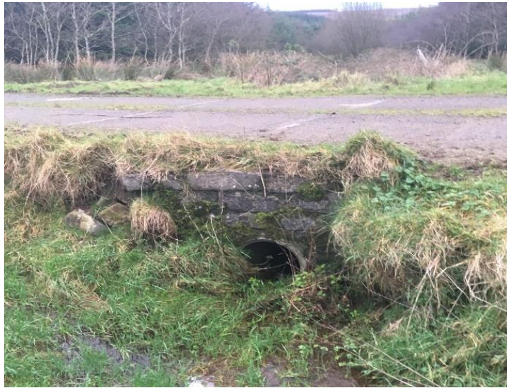
Watercrossing Structure W67
