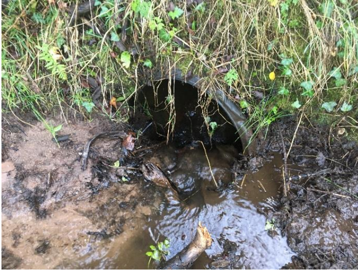
Watercrossing Structure W10
