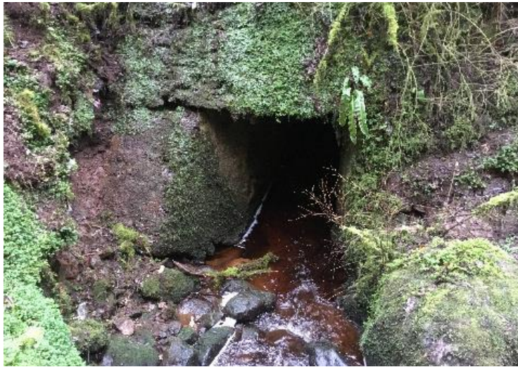
Watercrossing Structure W29
