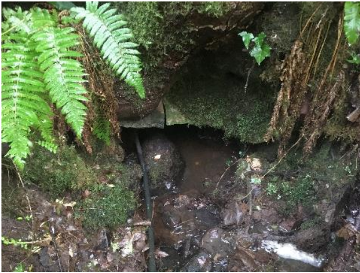
Watercrossing Structure W31
