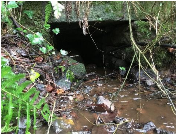
Watercrossing Structure W17
