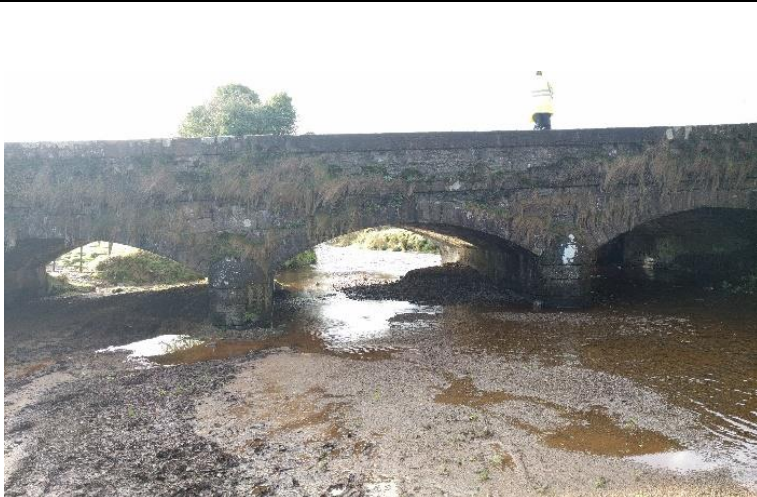
Watercrossing Structure W36
