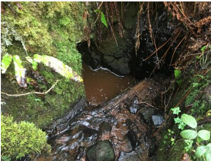
Watercrossing Structure W30
